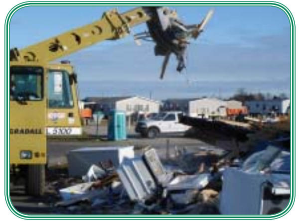
A GradAll picks up debris at Eastbrooke mobile home park.
