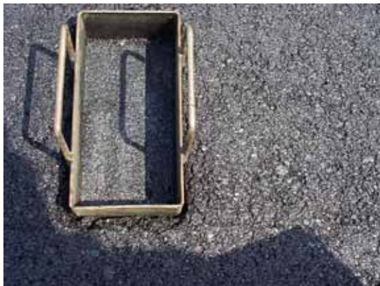
Template Placed in Asphalt Mat
